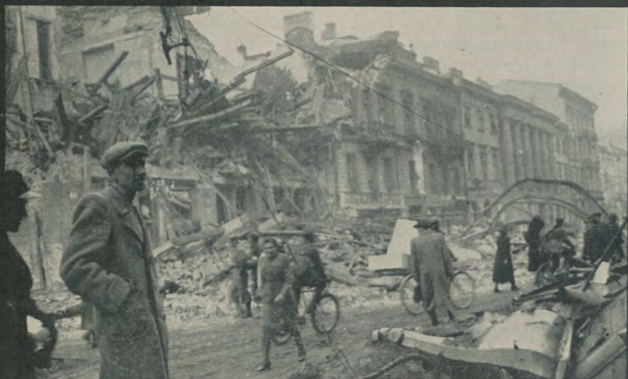
"New World Street," Warsaw's biggest business district, was a tangled mess of crumbled buildings and twisted trolley wires. Stunned civilians pick their way among the debris.
