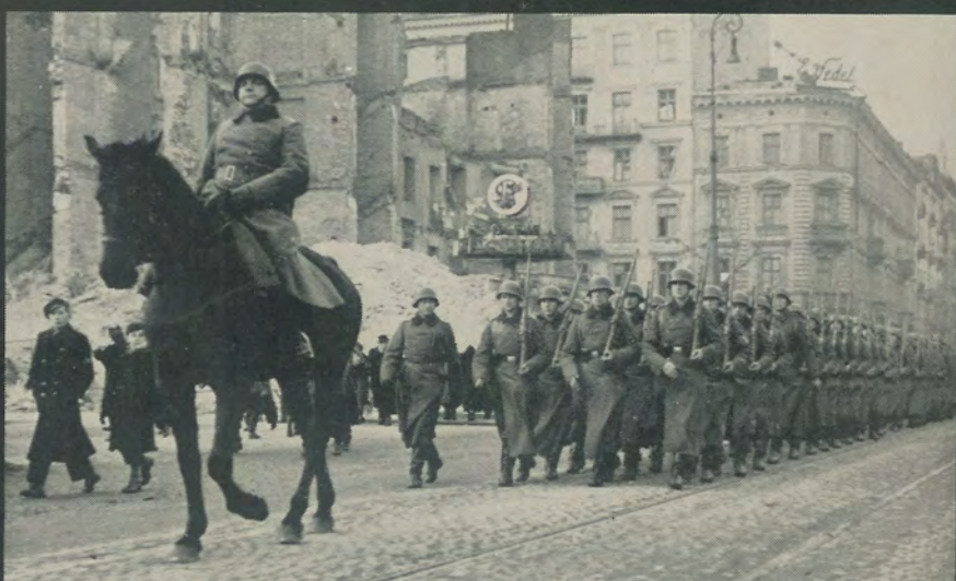
German troops marched into the city past the ruins of buildings on Oct. 1. These tall young shock troops are Hitler's finest. From Warsaw they were sent to Western Front.
