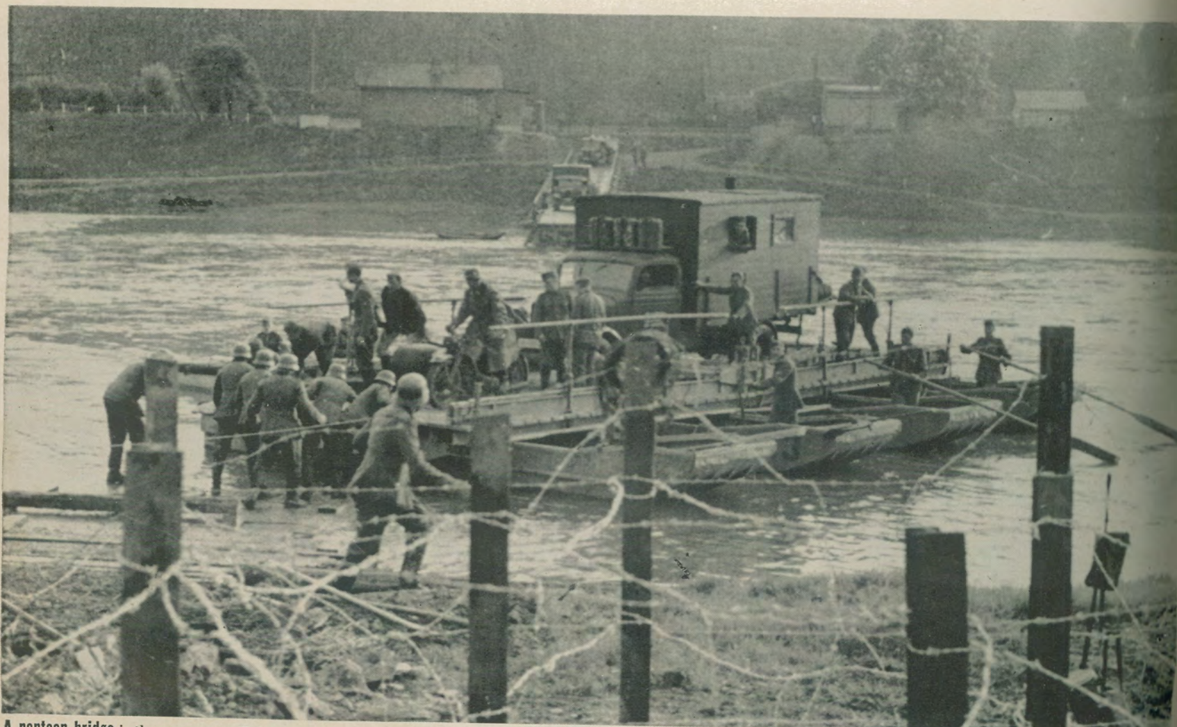
A pontoon bridge is thrown across a Belgian river by the Germans. The advance has stormed on past the barbed wire in the foreground. The engineers have completed the first section on the other side and here bring across with an
