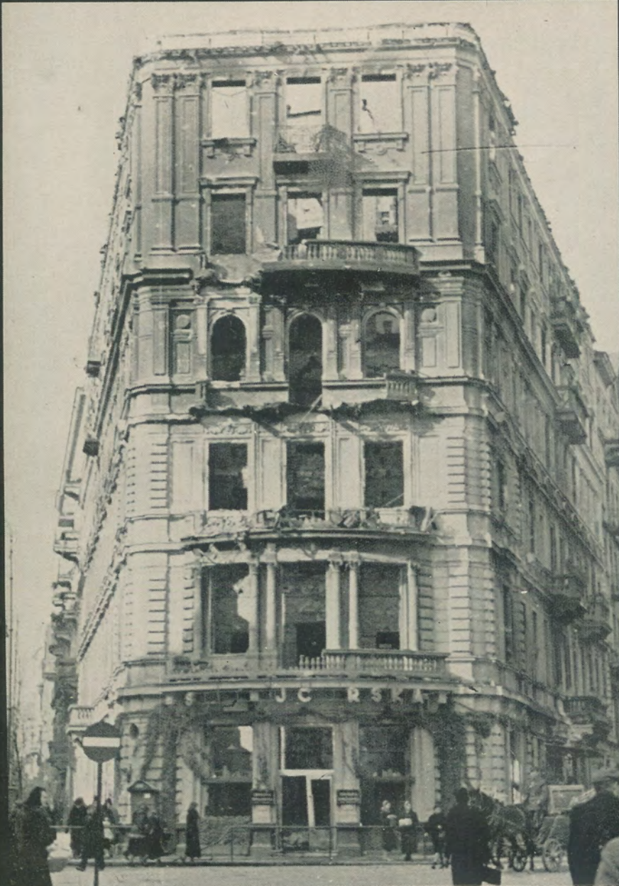
One bomb through six floors gutted this building housing official Gazeta Polska . All ruins over one story must be torn down in Warsaw to protect pedestrians from falling masonry
