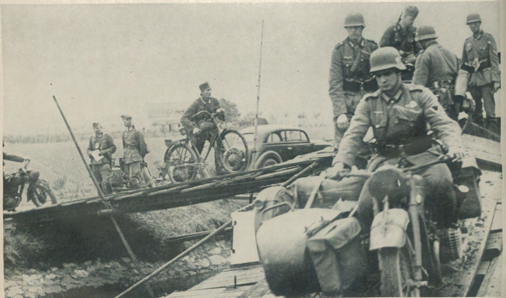
The army on wheels uses a large barge sunk in the Maas-Scheldt Canal as part of a bridge. The runway is made of barge hatch covers, and is braced with poles. An officer at the left directs the crossing while his staff car waits in cen-
