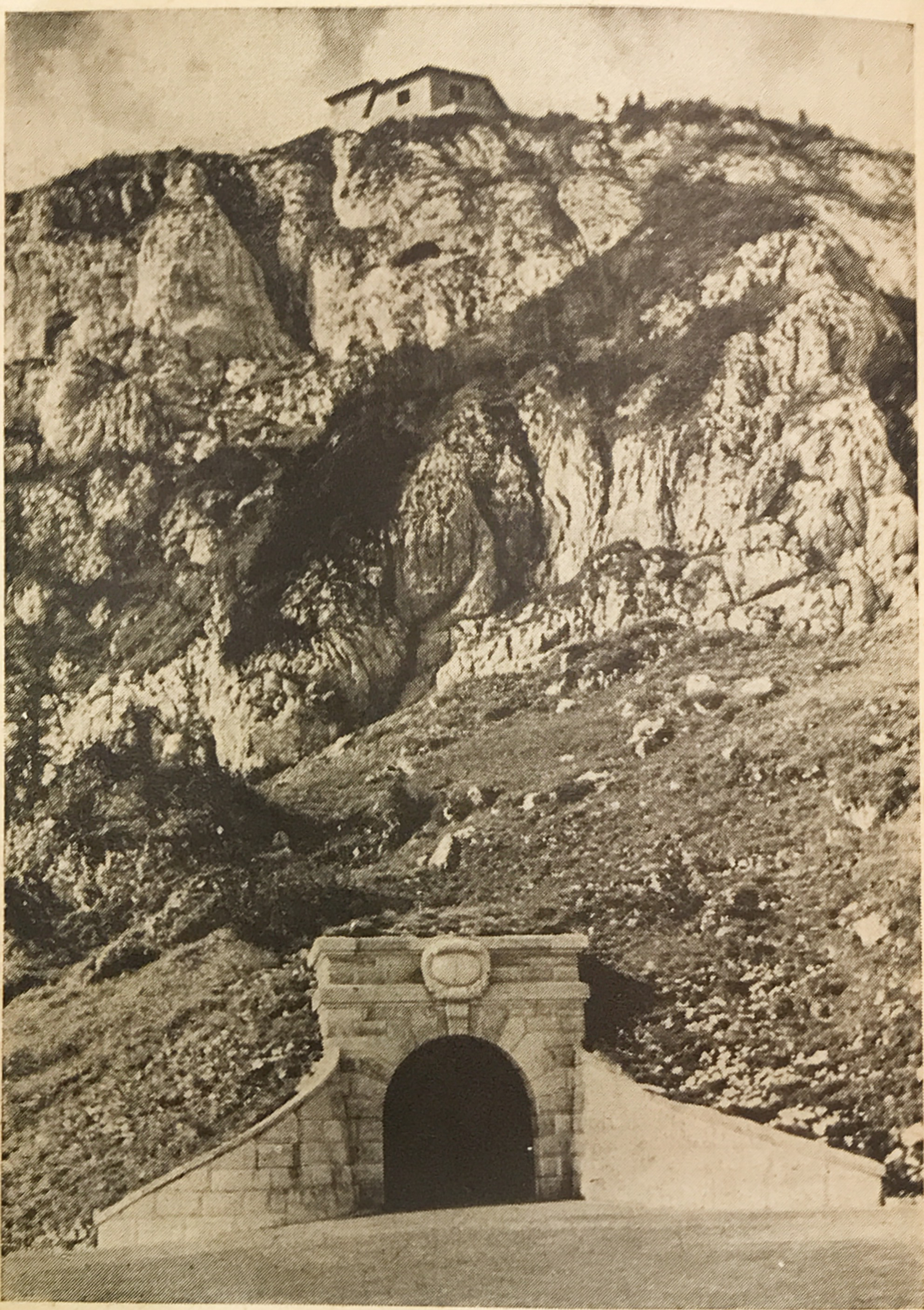
"Entrance to 140 mtr. - Elevator"
