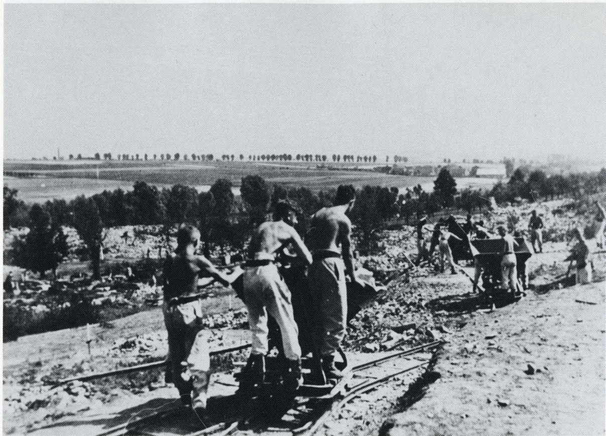
653. Clean-up of rubble of the destroyed village, Lidice, 1942.
